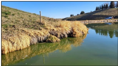
Figure 4 Erosional process in the southwestern shoreline of Cell 3.
