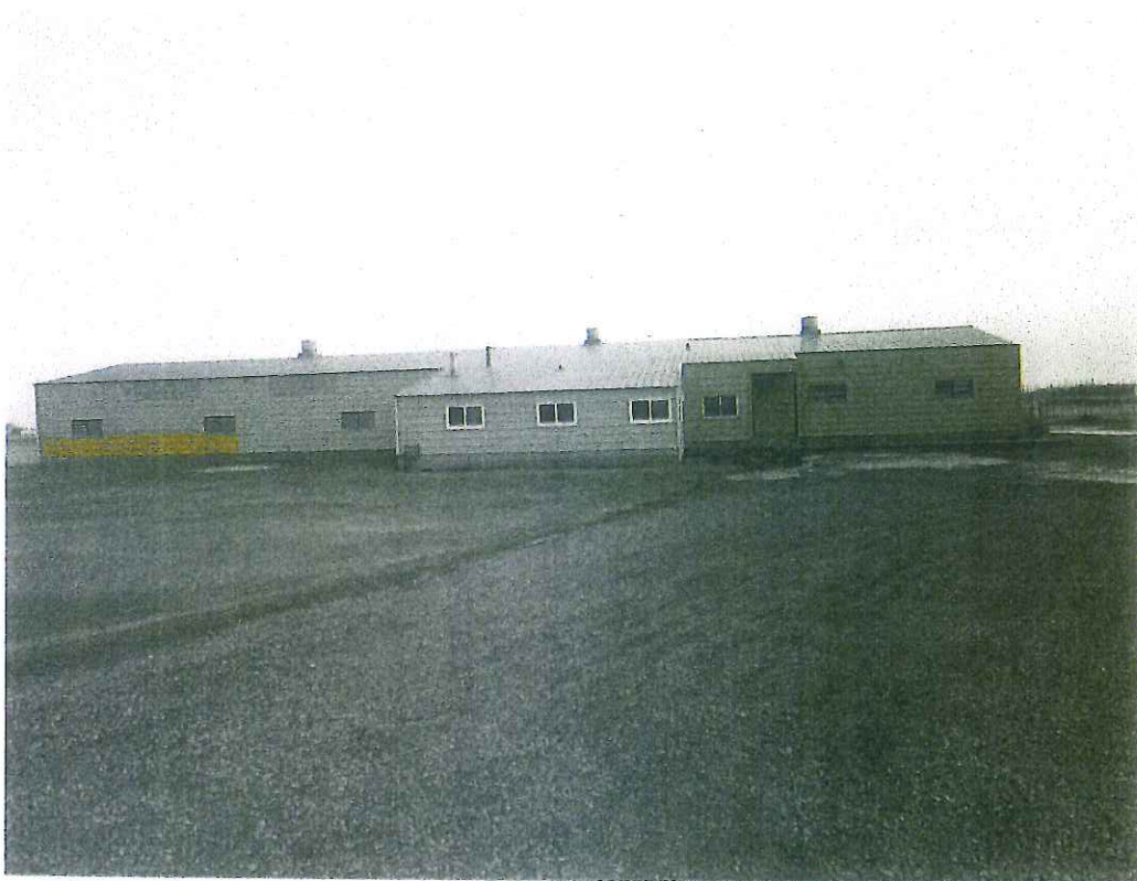
Photograph 1: Looking north across parking area at shop and office building constructed in 1982.
