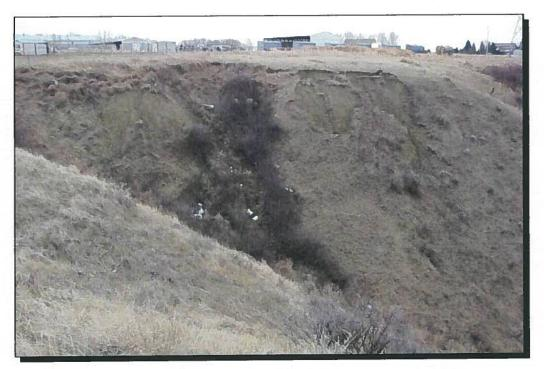
Photo 4 Skin Failures on North Perimeter Slopes (Looking South)
