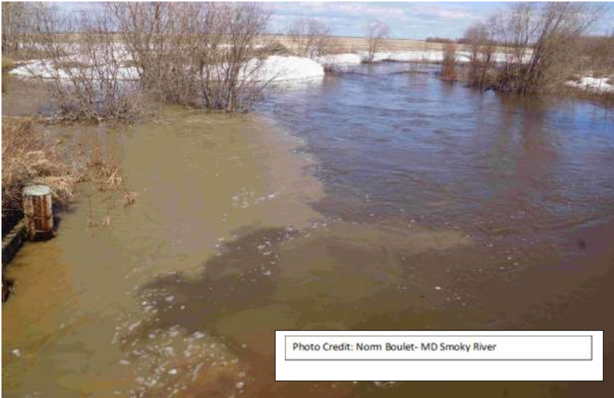
Picture 4: Brown water from road washout
