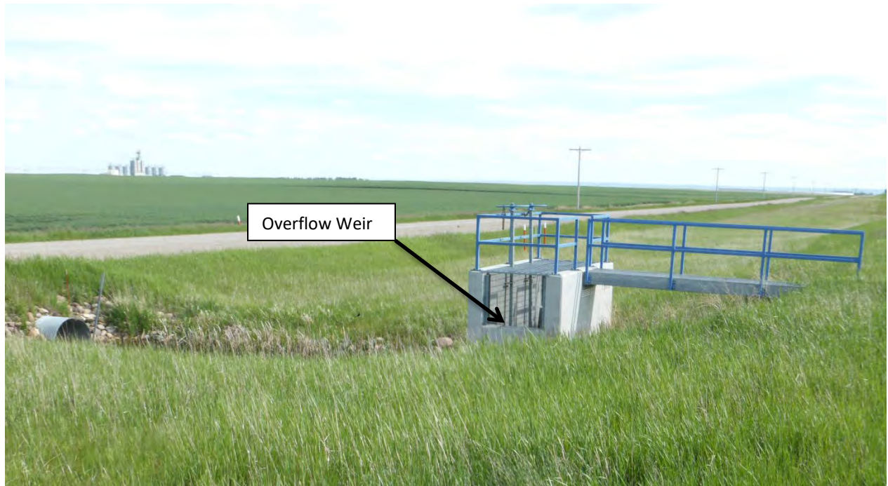
SMRID Main Canal Drain Inlet
