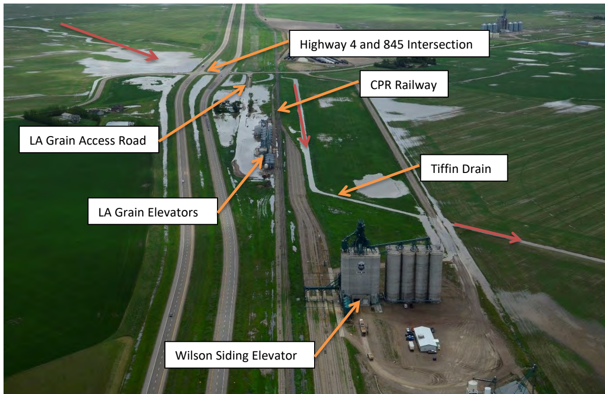
LA Grain Site Flooding June 19, 2014
