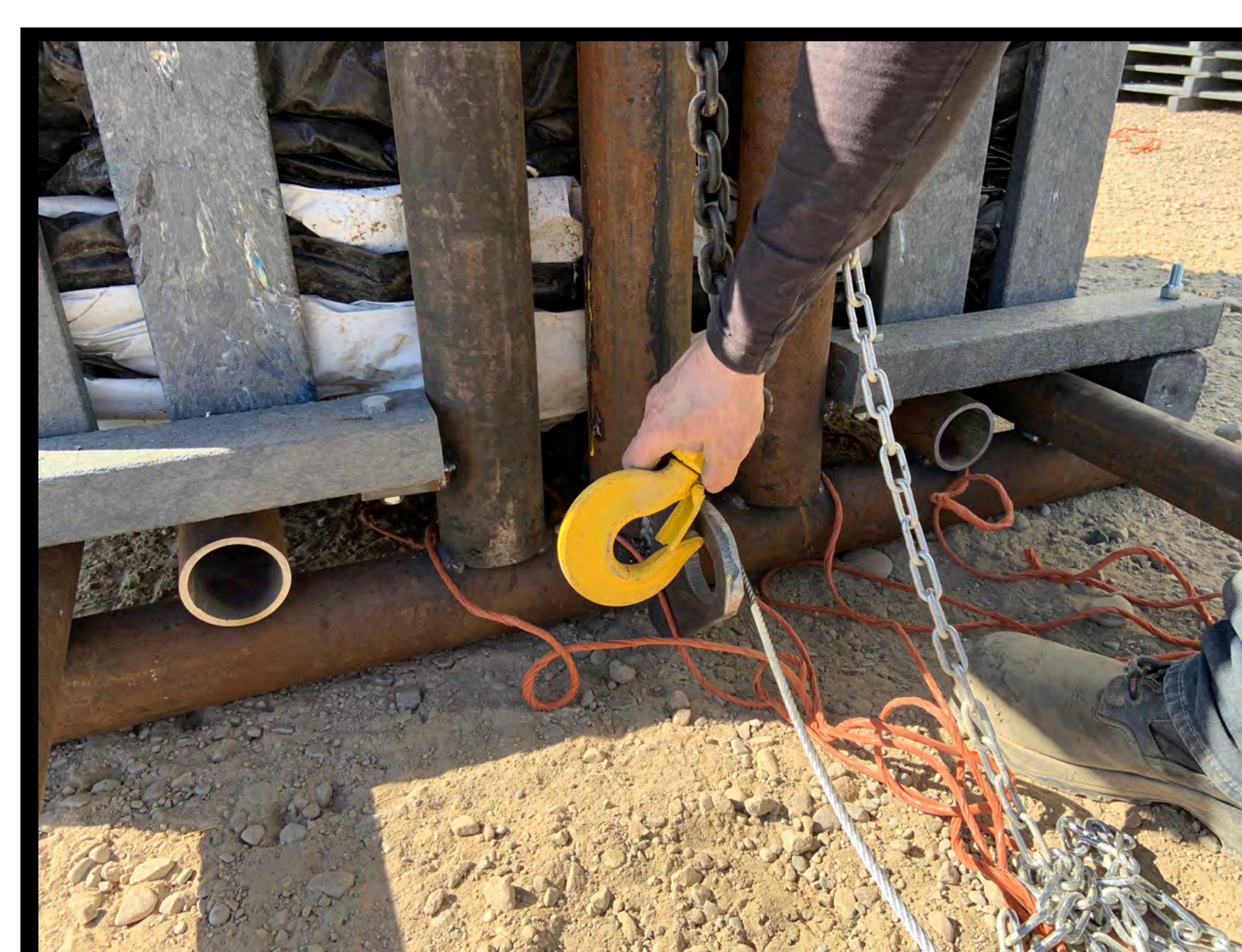
Disengage winch lock & attach hoist
