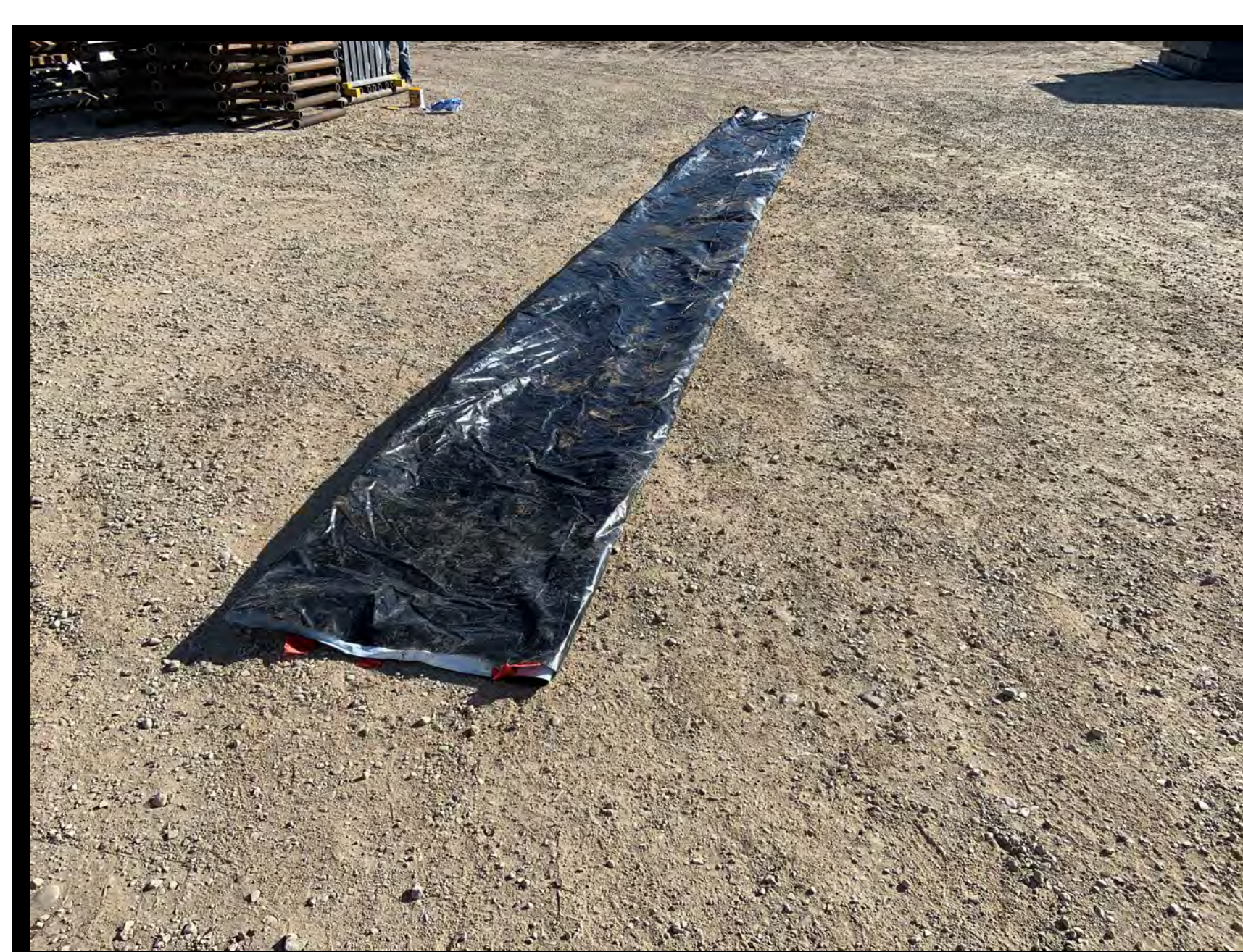
Fold sheets into 4' wide strips
